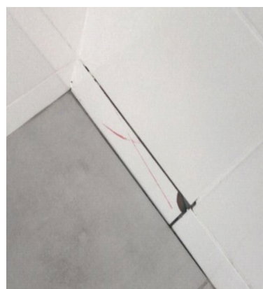
Figures 10 and 11. Pathological manifestations incidental to the ceramic coatings of enterprise A
