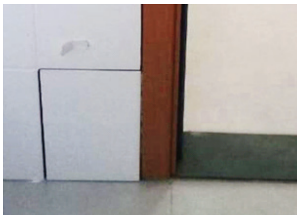
Figure 16. Lack of grout found in surveys at enterprise B
